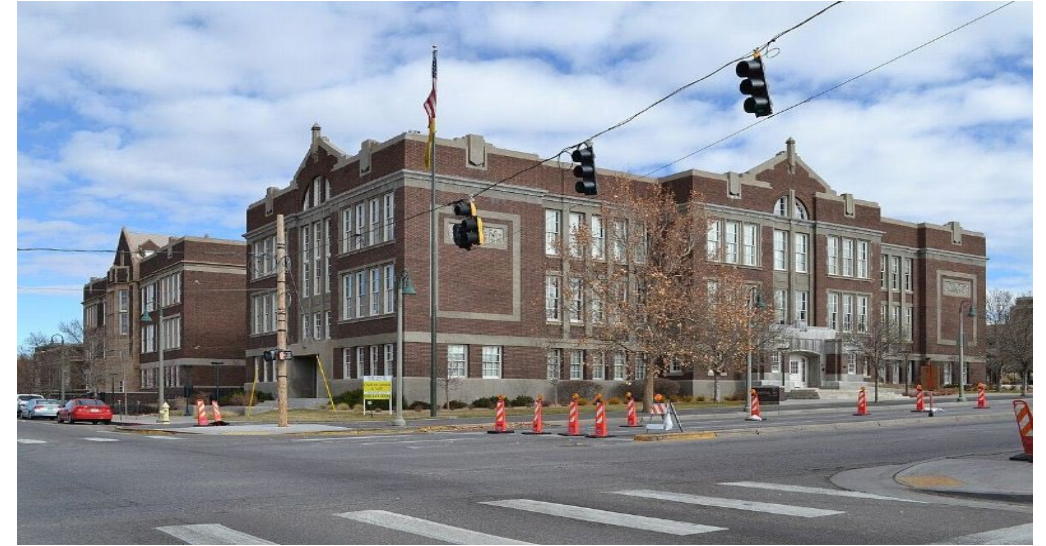
Old high school building
