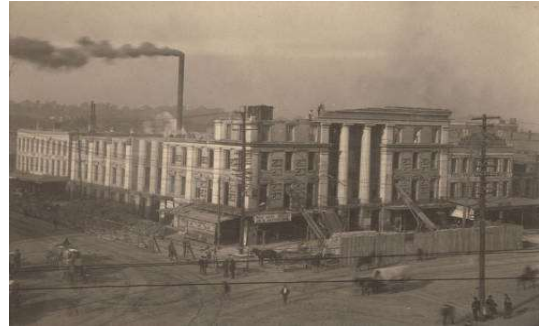
Picture 4: Demolished old hotel for new one
